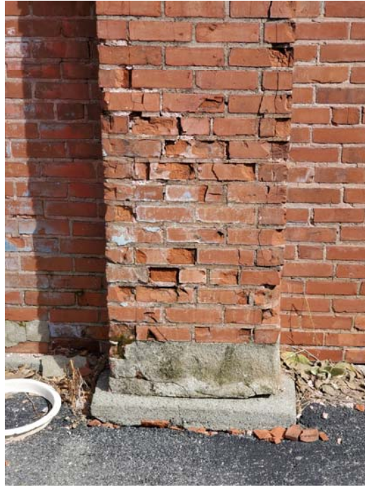
Photograph #15 – Deteriorated Exterior Masonry
