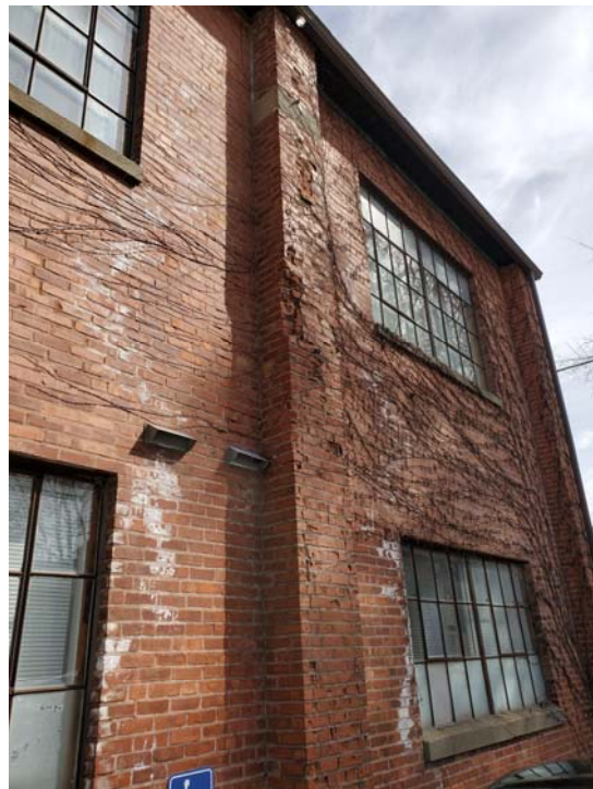
Photograph #16 – Deteriorated Exterior Masonry
