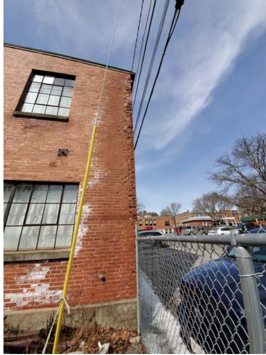
Photograph #17 – Deteriorated Exterior Masonry
