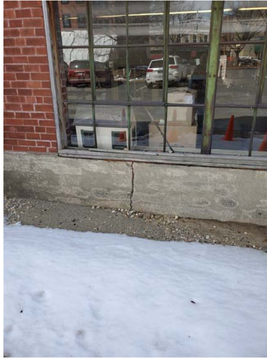
Photograph #19 – Cracked Foundation Wall
