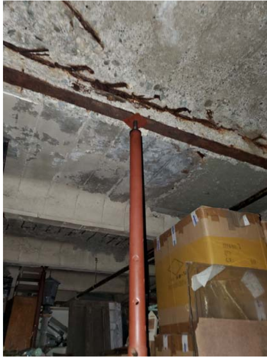
Photograph #9 – Temporary Shoring Post Below Spalled Concrete Joist
