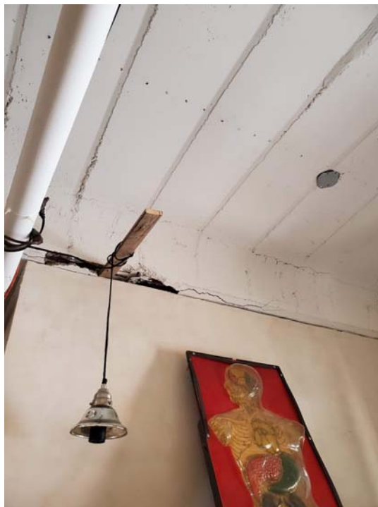
Photograph #5 – Spalled Concrete Joist
