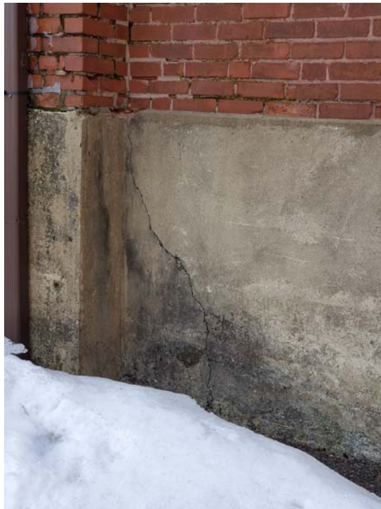
Photograph #18 – Cracked Foundation Wall
