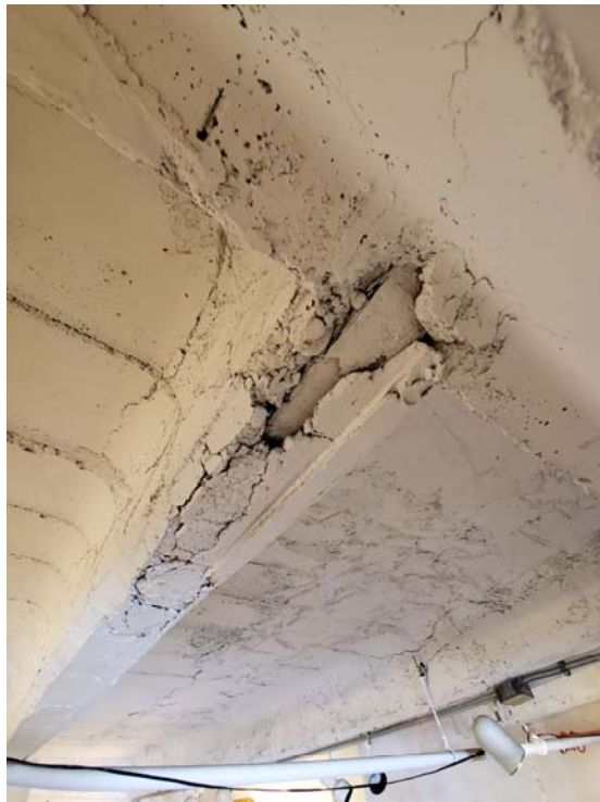
Photograph #8 – Spalled Concrete Joist
