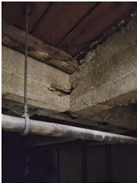
Photograph #1 – Spalled Concrete Along Concrete Beam
