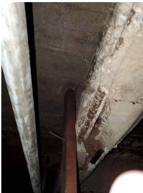
Photograph #2 – Spalled Concrete Along Concrete Beam
