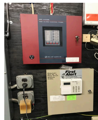
Fire Alarm Control Panel
