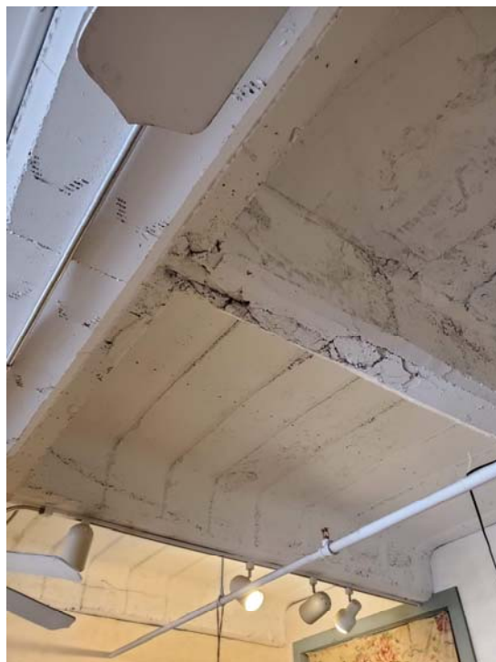
Photograph #4 – Cracked & Spalled Concrete Joist
