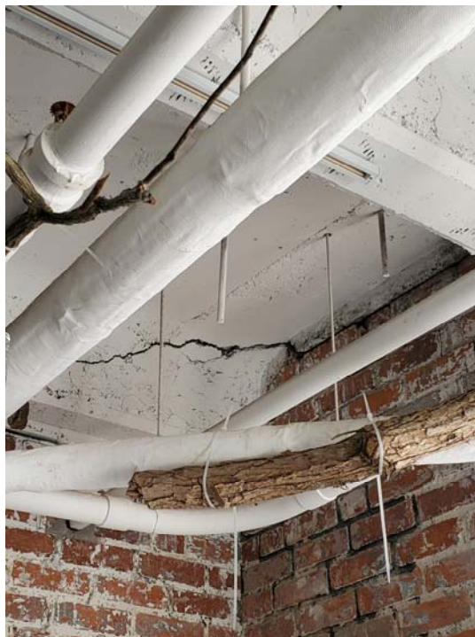
Photograph #3 – Cracked Concrete Joist
