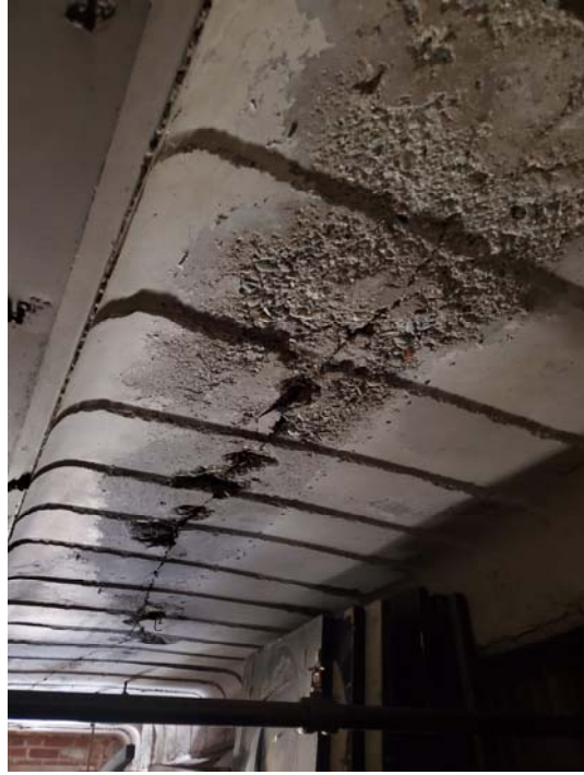
Photograph #11 – Cracked Concrete Slab
