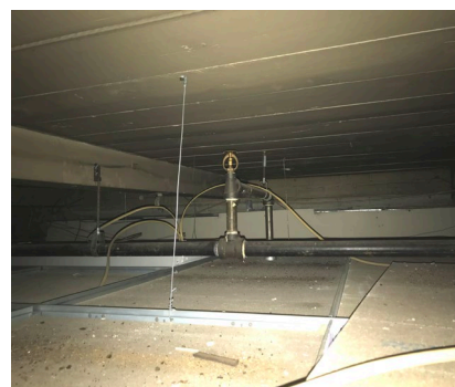
Sprinklers Above Ceiling
