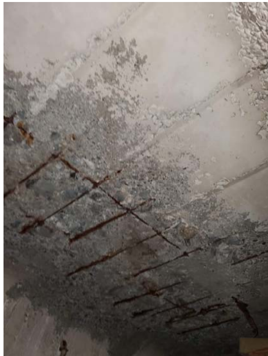
Photograph #10 – Spalled Concrete Slab
