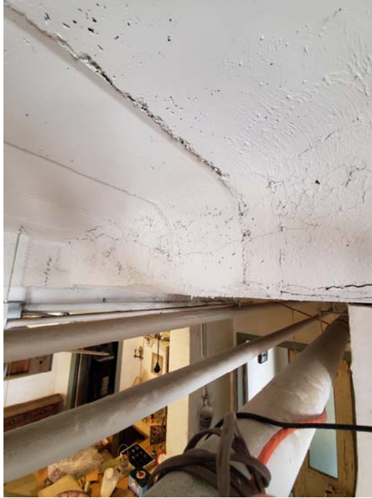
Photograph #7 – Hairline Cracks in Concrete
