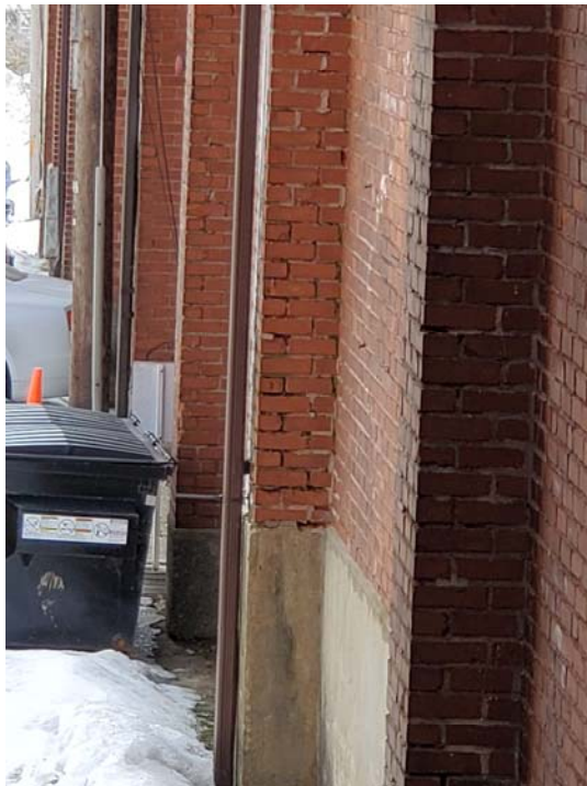
Photograph #12 – Deteriorated Masonry Joints
