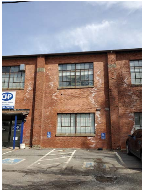
Photograph #14 – Exterior Masonry Efflorescence
